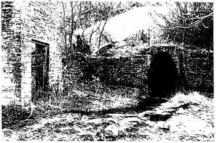
Figure 2: The portal of the Blackett Level, Allendale, Northumberland UK, in 1997. Driven between 1854 and 1896, the level still flows at up to 20 Ml.d<sup>-1</sup>, permanently dewatering mines up to 7 km away.
