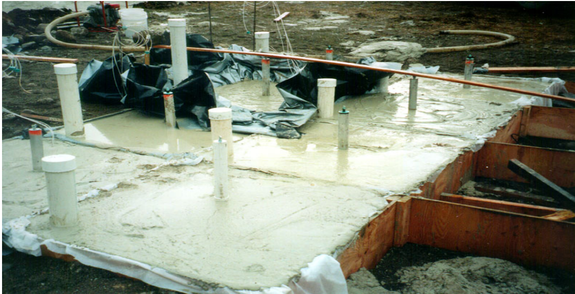
Figure 6 – Construction of field paste cells.
