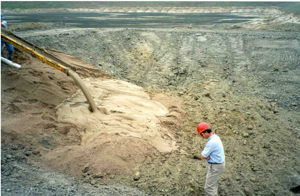
Figure 1 – Paste placement. Note the absence of any free water despite low viscosity.
