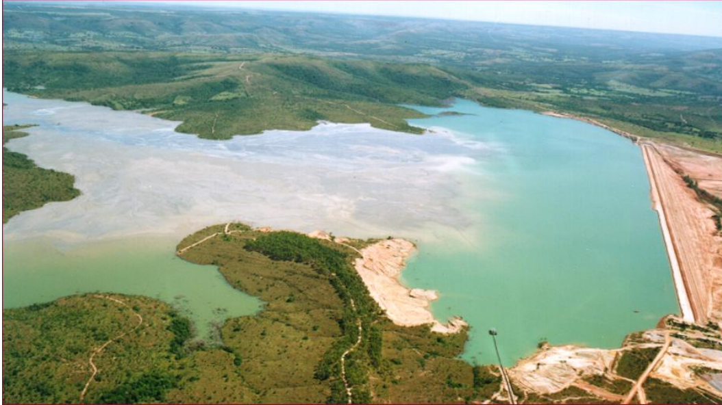
Figure 5: Tailings dam facility
