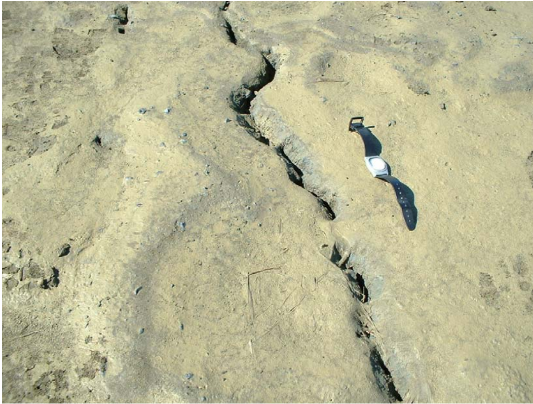
Figure 7. Cracks on the Co-Mix cover of Cell #5.
