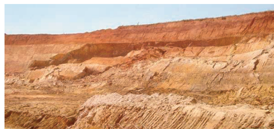
Fig. 1 Rotational slide failure of Pit 2 walls at the mine site. Photo taken during dry season.
