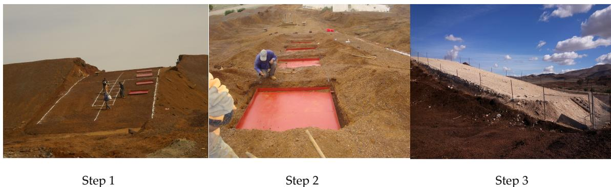
Figure 2 Photos illustrating the field inclined SR cover construction steps
