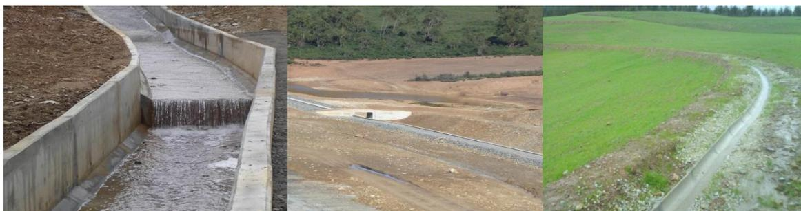
**Figure 7** Aljustrel cleanwater diversion channel and Vale d'Abrutiga surface run-off drainage system.
