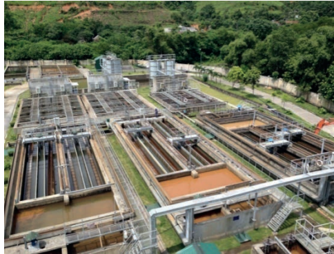
Figure 4 VangDanh MWTP: capacity of 3,000 m 3 /h, designed with 3 treatment lines
