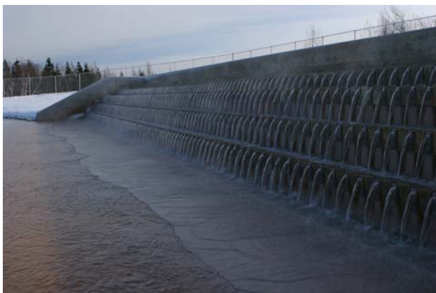
Fig. 2 Cascade at the newly constructed passive mine water treatment system of the IB hydraulic system on Cape Breton Island, Nova Scotia, Canada
