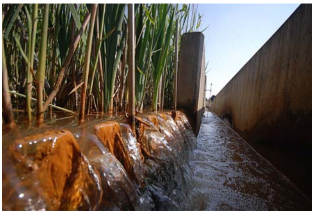
Fig. 3 Mine water treatment in a British reed bed (photo: Dave Johnston; Mine waters Technical Advisor, Environment Agency)
