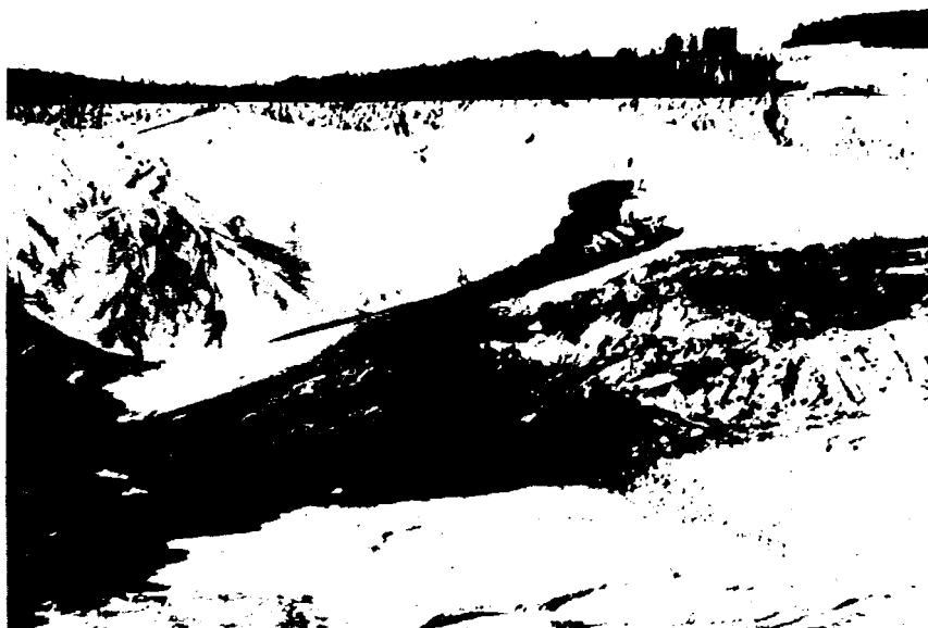
FIGURE 15 - PIPING AT DOWNSTREAM FACE OF SAND TAILINGS DYKE.
