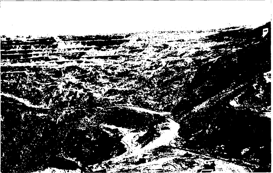
JEFFREY MINE FIGURE 8: SLIDE AREA FROM WEST
