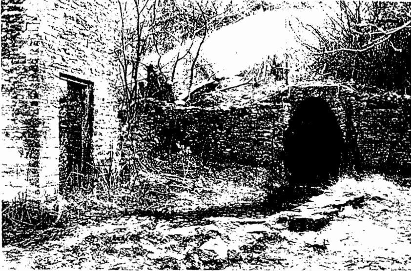
Figure 2: The portal of the Blakett Level, Allendale, Northumberland UK, in 1997. Driven between 1854 and 1896, the level still flows at up to 20 Ml.d<sup>1</sup>, permanently dewatering mines up to 7 km away.
