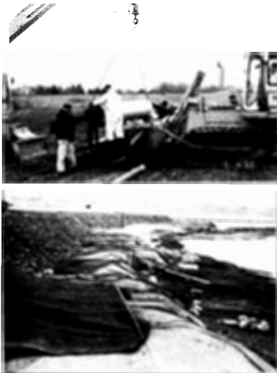
Figures 14 and 15. Preparation and placement of sand mats.
