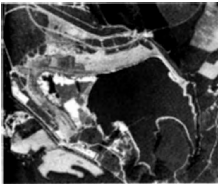
Figure 6: Aerial view of the Helmsdorf TMF.
