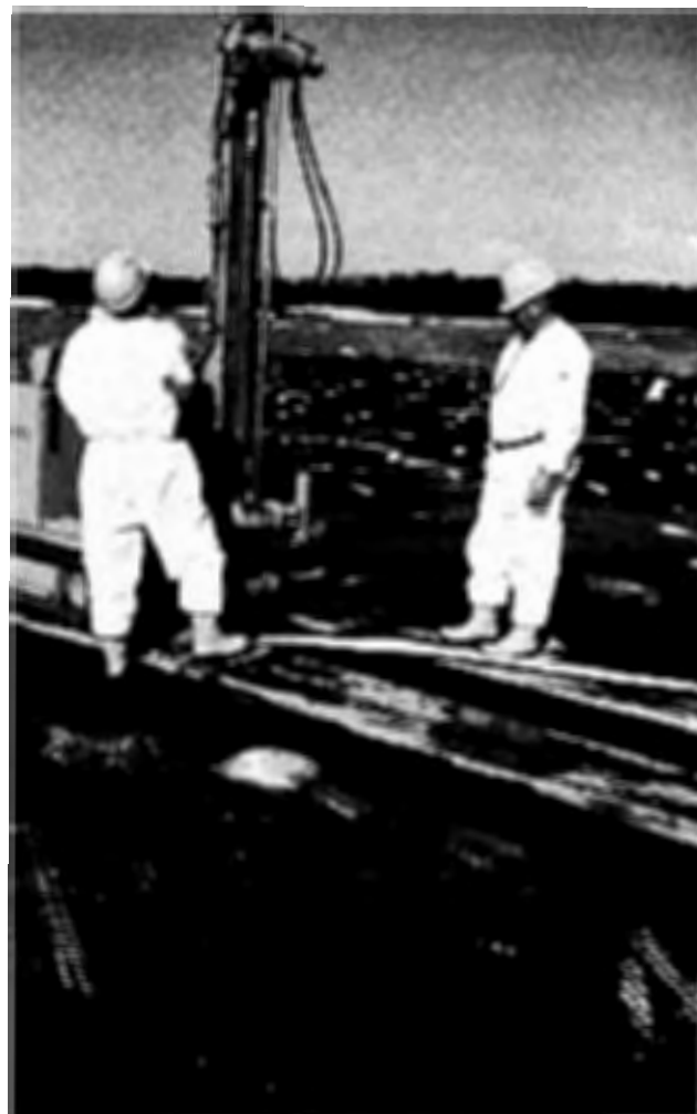
Figures 12 and 13. Installation of vertical wick drains.
