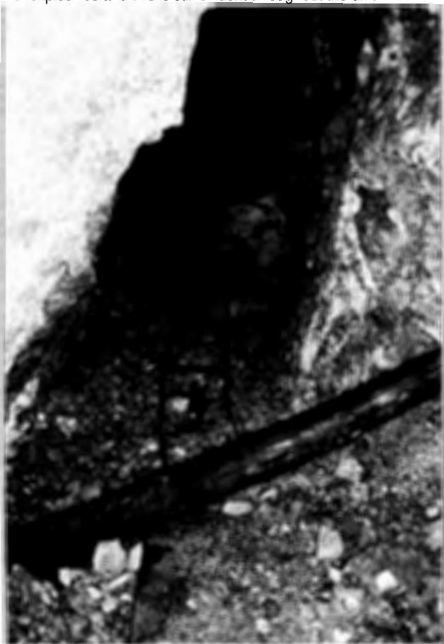
Figure 5. Section leading from the main drift to the well, at the end of the tracks. This is where the ventilation hole is found.
