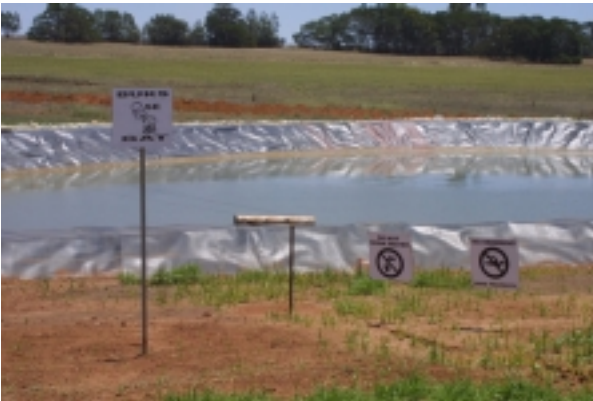
Figure 2. Temporary dam constructed to store water at Buks se Gat.
