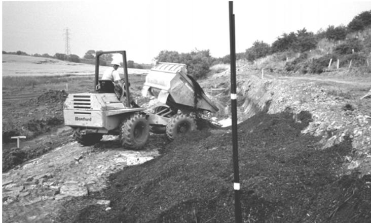
**Figure 4 Construction of the PRB at Shilbottle, Northumberland.**
