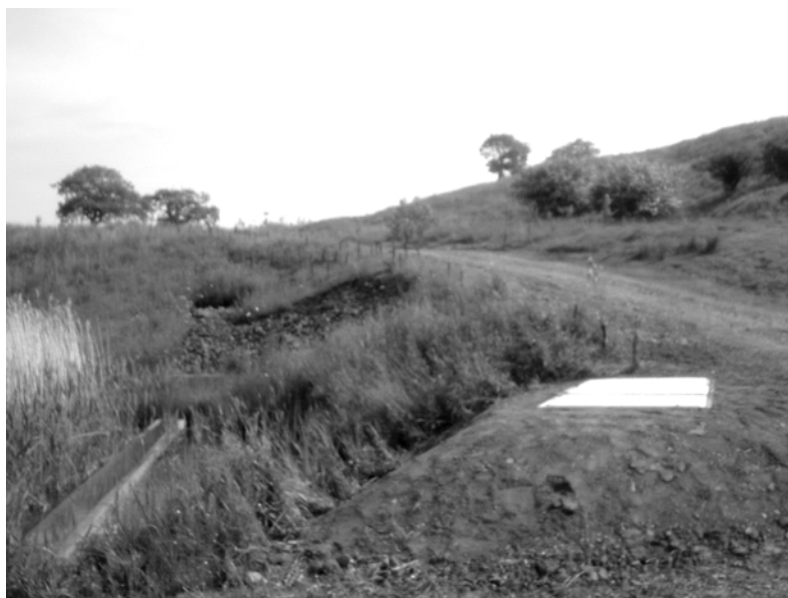
Figure 2: The manganese treatment system in place at Whittle treatment wetlands, Northumberland, UK.
