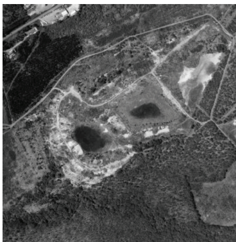
Figure 2. Tailings pile with free water on the top.
