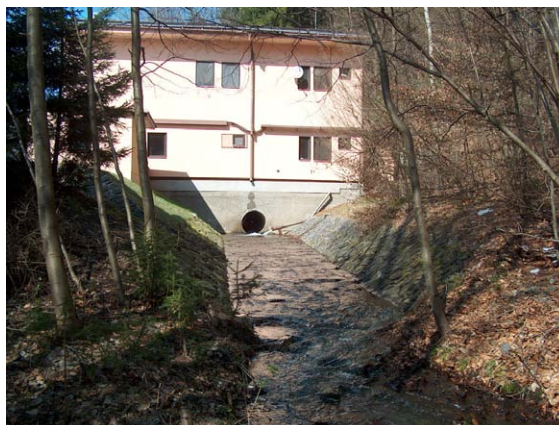
Figure 1a Photos of the discharge pipe and the building of the MWTP on the Hadůvka stream
