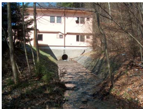
Figure 2. Photos of the discharge pipe and the building of the MWTP on the Hadůvka stream
