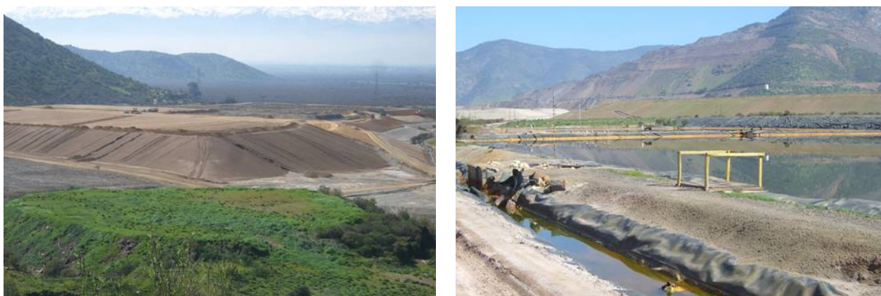
Figure 6. rock pile at Lo Aguirre site during mine closure (left) and basins for collection and evaporation of leachate (right)
