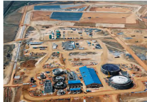
Construction of Optimum Water Reclamation Plant - September 2009
