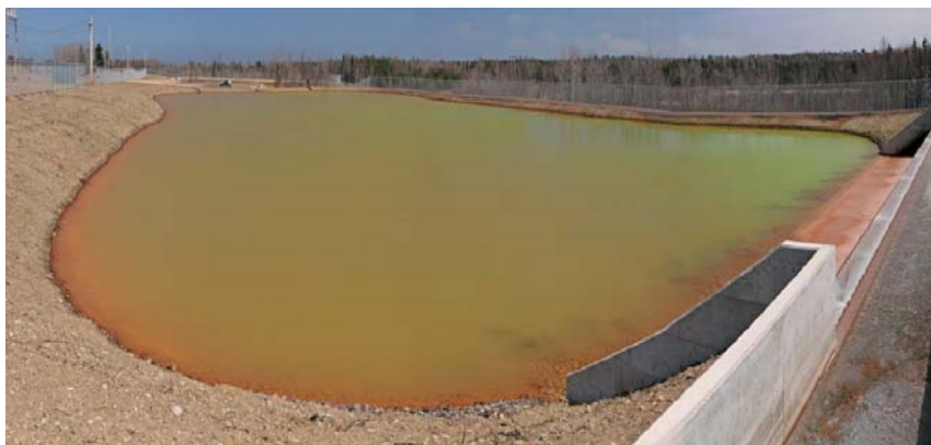
Figure 1 View of the Neville Street settling pond with the mine water inflow and cascade on the right and the outflow in the upper left corner. Length of the settling pond 150 m, width 60 m
