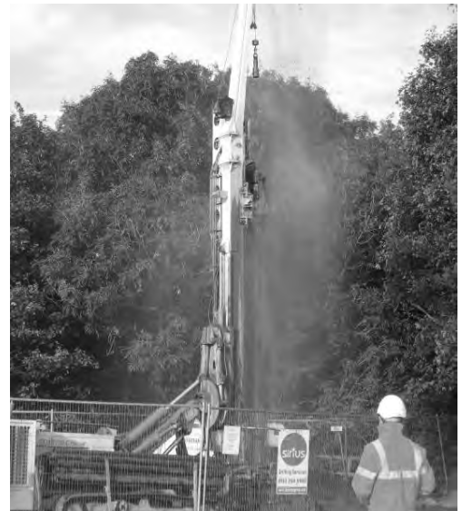
Plate 1 Air lift purging of North OBS BH.
