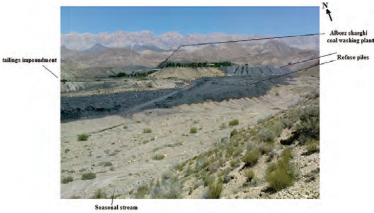
Figure 1 View of the Alborz Sharghi coal washing plant, coal refuse piles and tailing impoundment.
