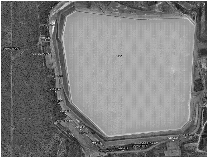
Figure 1 Locations of Drilling Investigations / Monitoring Bores (South and West Wall areas)
