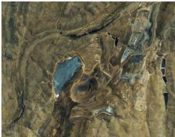
Figure 1 Mine tailings nearing capacity
