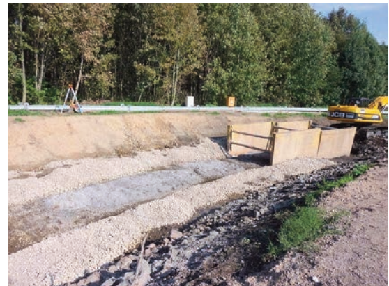
Fig. 7 Before (left) and during (right) the exchange of the riverbed material
