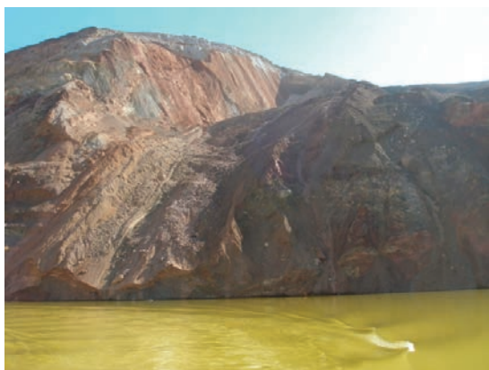
Fig. 3 A landslide covering several pit benches.
