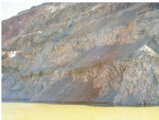
Fig. 2 Rock spall on pit benches.
