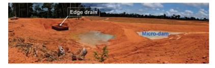
*Fig. 6 Micro-dam built on drainage channel.*
