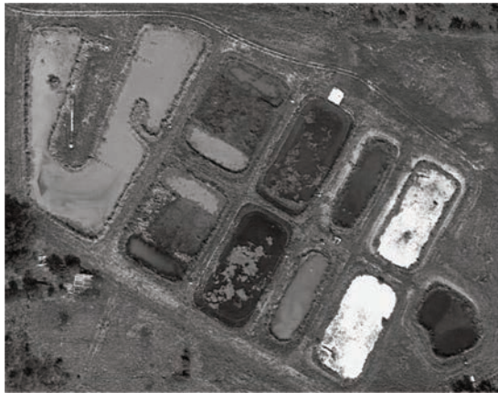
Fig. 1 Mayer Ranch passive treatment system, Tar Creek Superfund Site, Oklahoma, USA.
