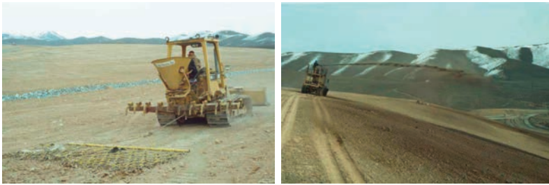
Fig. 3 AA Leach Pad plant seeding (left) and organic mulch application (right).
