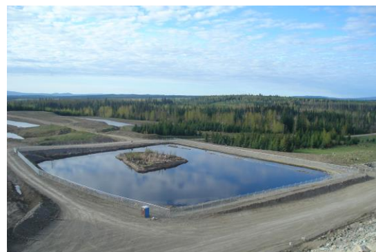
Figure 2 View of the completed BCR looking down from the top of the tailings storage facility.
