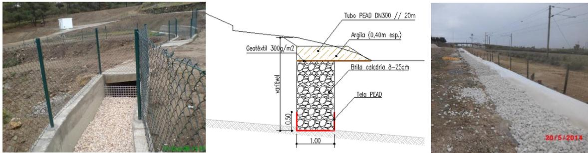
**Figure 8** Mine gallery open limestone drain (left) and anoxic limestone drain before soil cap(center and right).
