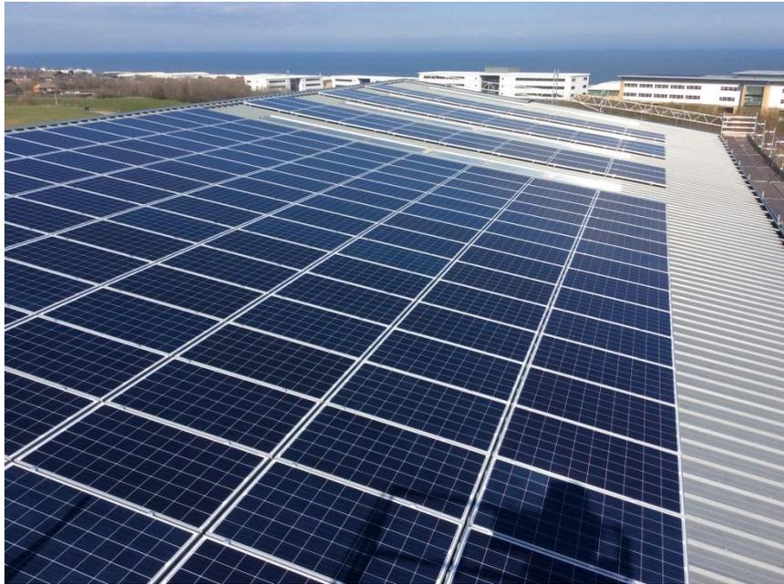
*Figure 1 Dawdon active scheme 49.92Kw scheme installed in 2016 consisting of 192 260 W panels.*
