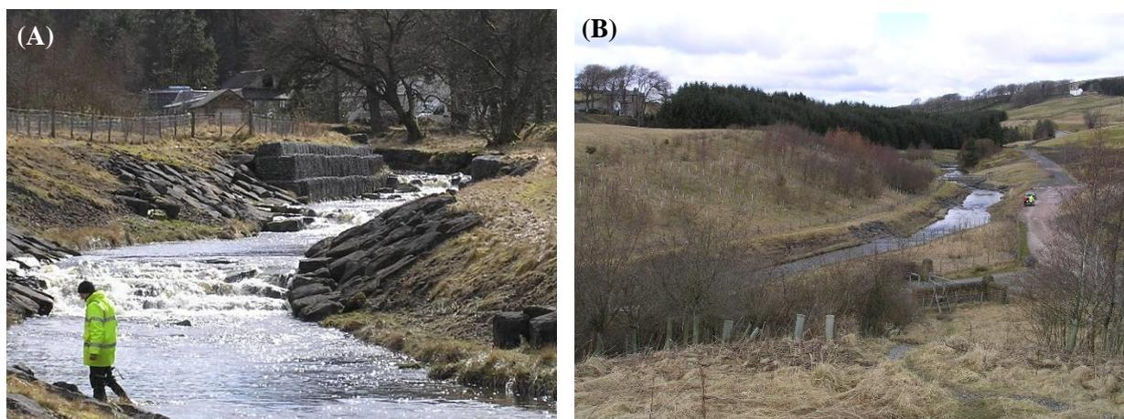
**Figure 2.** Use of gabions to stabilise banks of the River Nent, Cumbria (A) and re-grading, capping and vegetation of spoil material along the same stretch of river (B)
