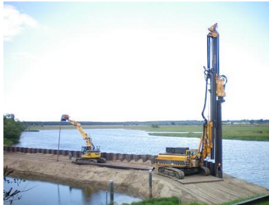
Figure 15: Construction of a ship lock near Quitzöbel , Germany. Sheet pile installation with RTG RG 19T and Top Vibrator MR 105 V
