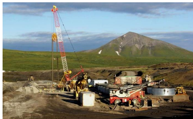
Figure 14: Cut-off wall installation with cutter BC 40
