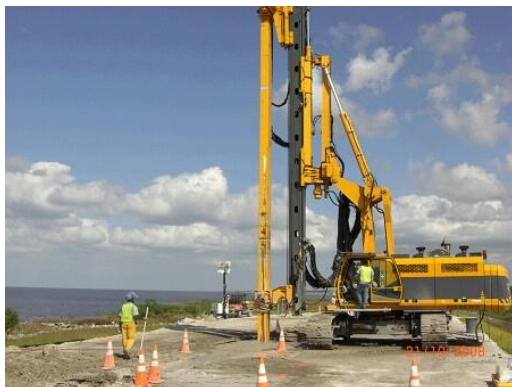
Figure 11: CSM installation with RG 25 S
