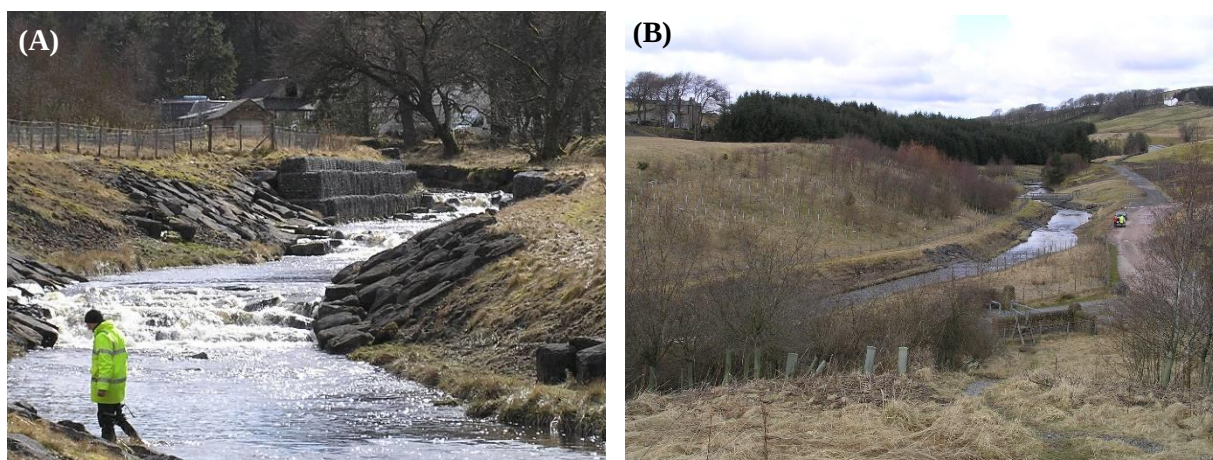
Figure 2. Use of gabions to stabilise banks of the River Nent, Cumbria (A) and re-grading, capping and vegetation of spoil material along the same stretch of river (B)
