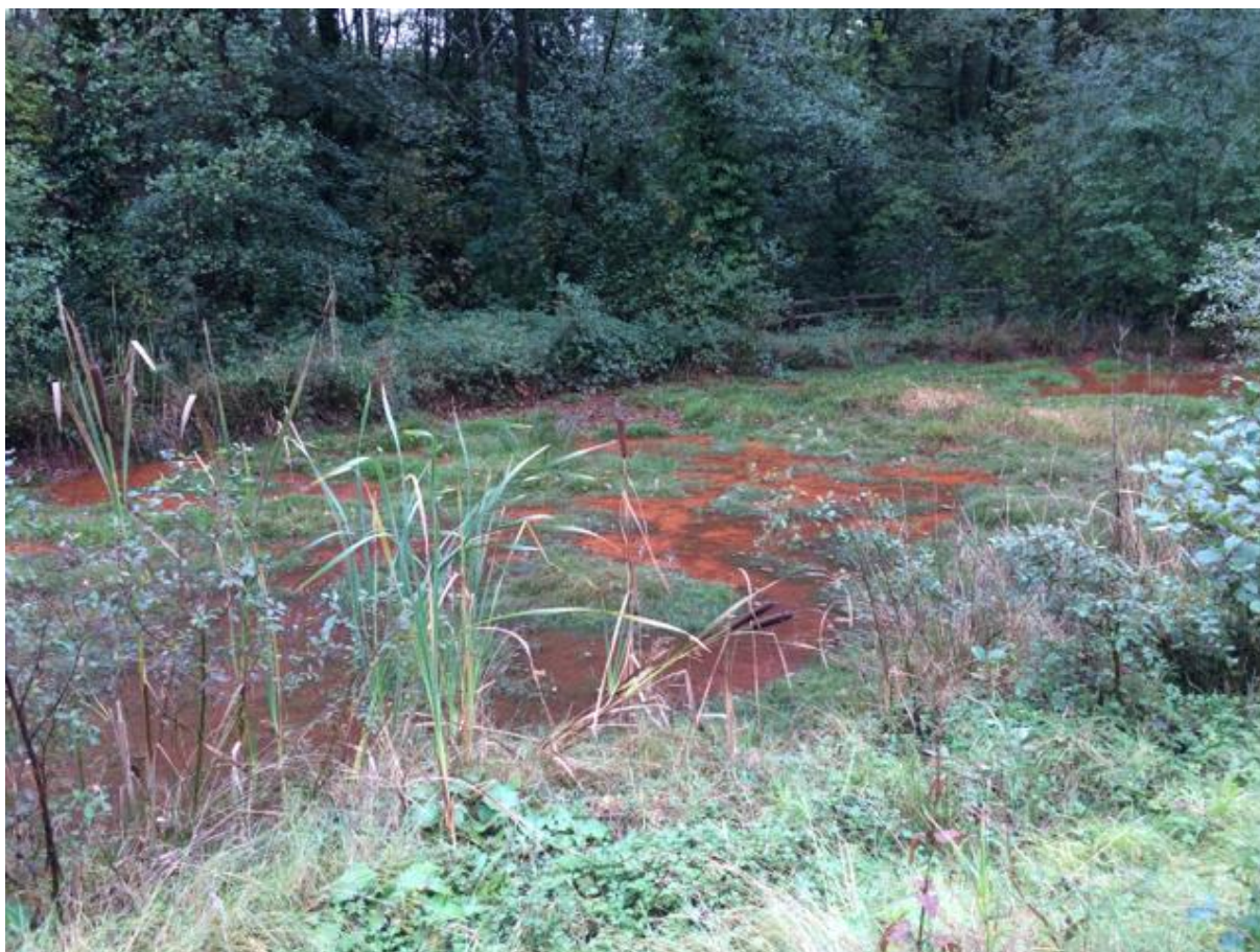
Figure 1 Photograph of Tan-y-Garn RAPS; note accumulation of HFO at the surface and vegetation growth
