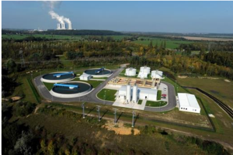
Figure 4 MIBRAG Mine water treatment plant.
