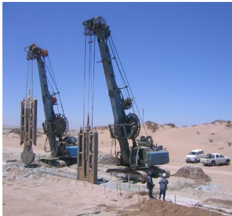
Figure 8: Cut-off wall installation BAUER GB 60
