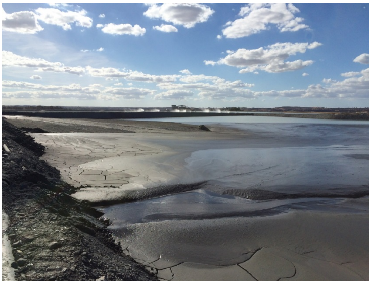
Figure 4 Operational Paste Placement.
