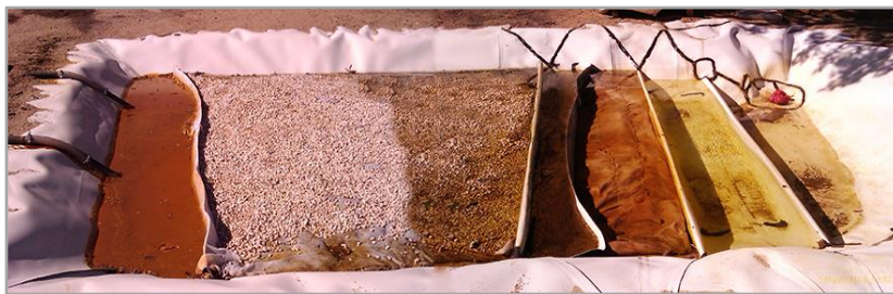
Figure 3 Mine water passive treatment pilot plant
