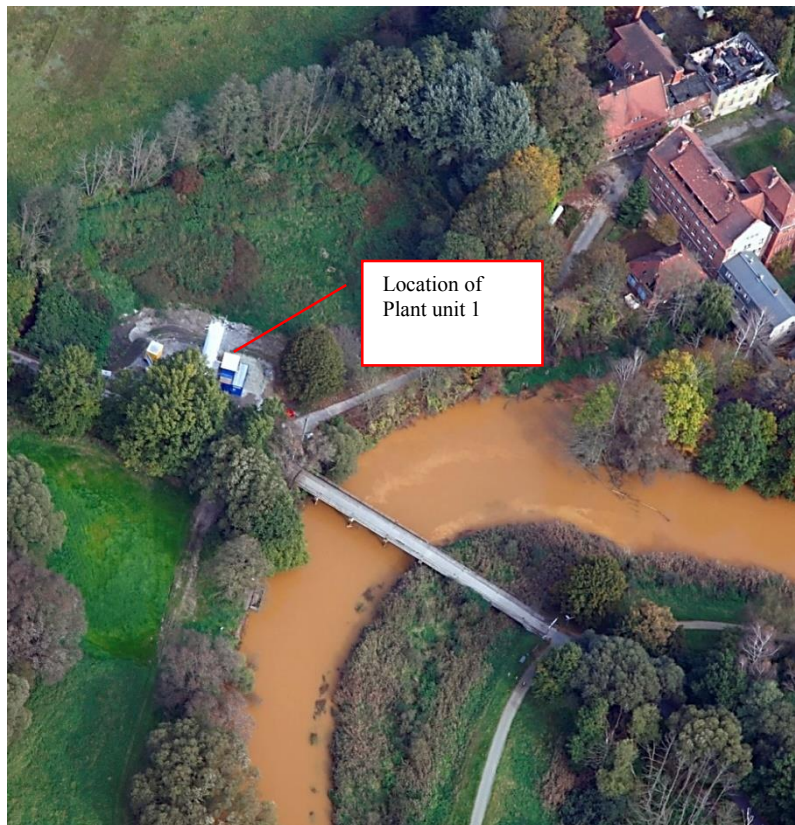
Figure 1 View of plant unit 1 in Spremberg Cantdorf and in-stream lime dosing
