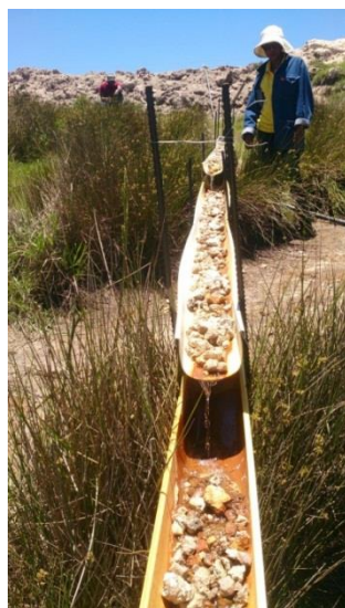
Figure 3 Carolina pilot passive treatment cascading trench
