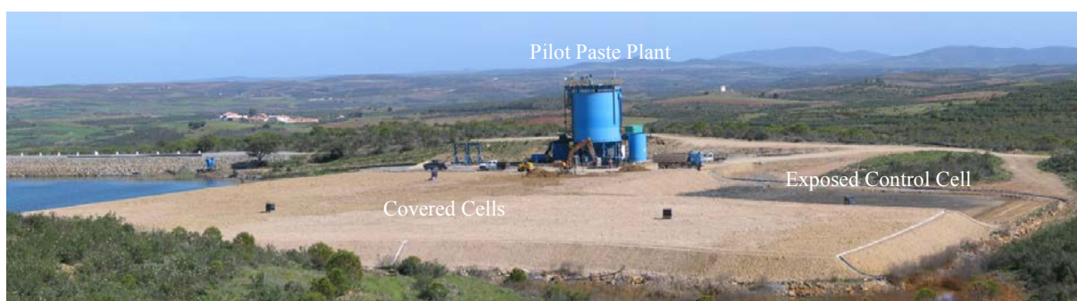
Figure 3 Paste Trial after Construction.
