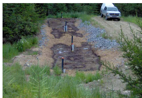
Figure 2 Passive treatment system on Lorraine mine site, Quebec, Canada.
