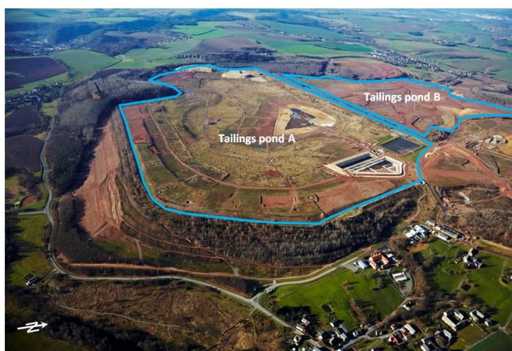
Figure 1 Tailings management facility (TMF) Culmitzsch, Seelingstädt, Germany (November 2015).
