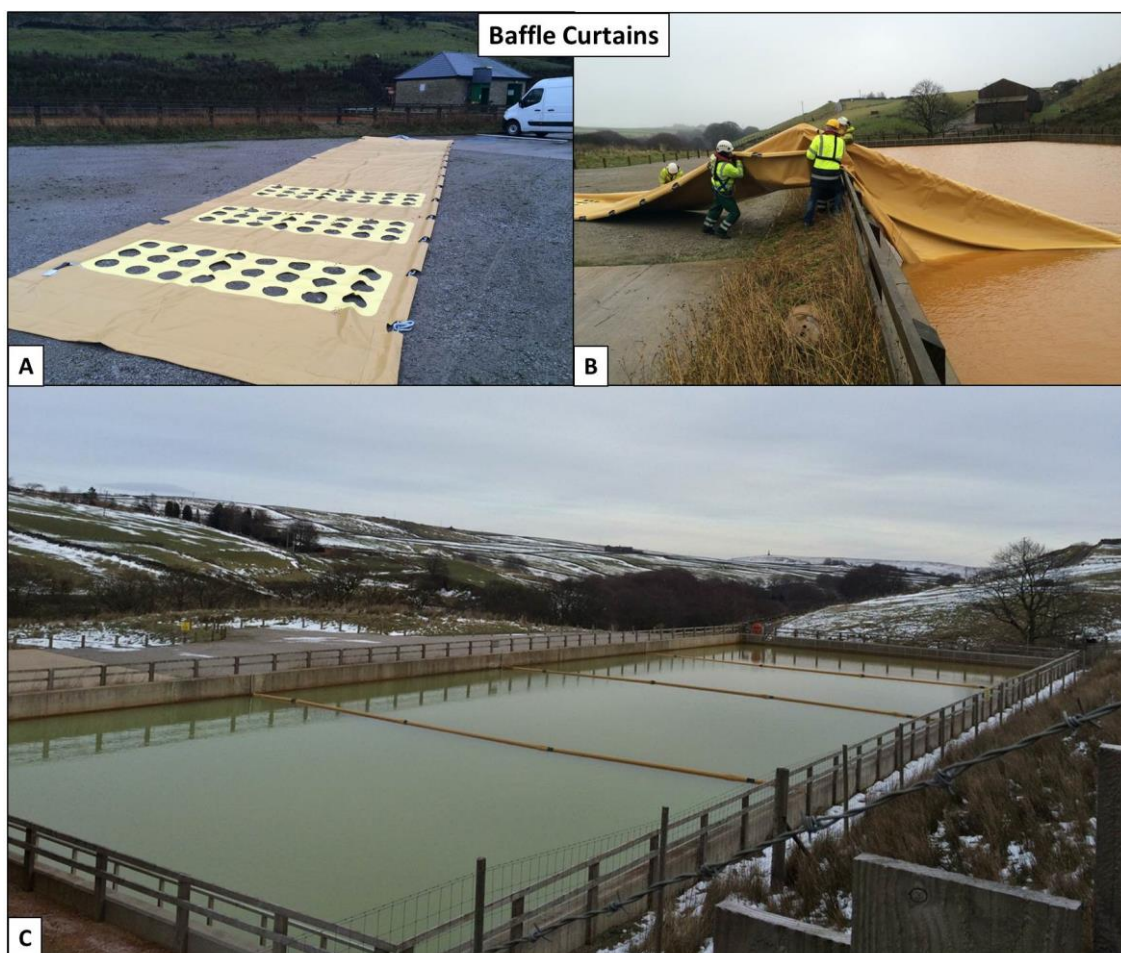
Figure 2 – Baffle Curtains; A) Baffle curtain prior to installation B) Retrofitting of the baffle curtains C) Baffle curtains after installation
