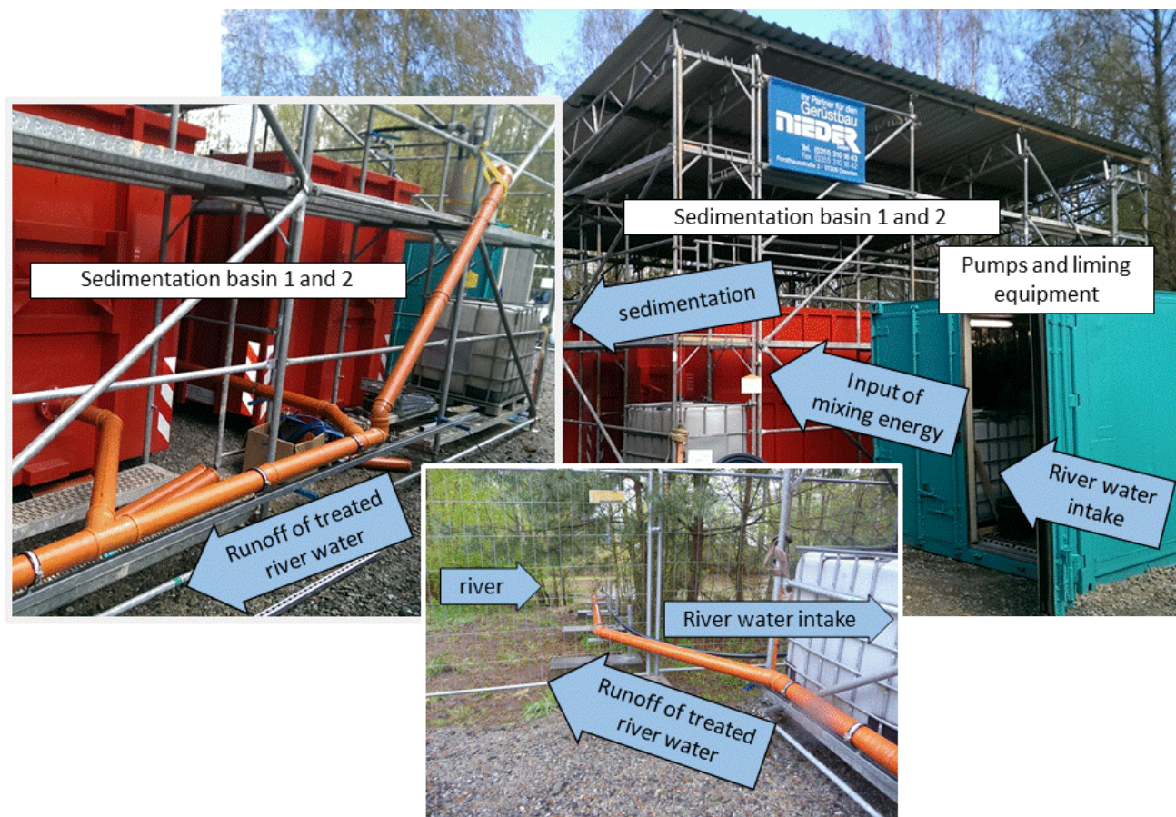
Figure 2 Pilot plant in the field to test various combinations of mixing, liming and sludge recycling.
