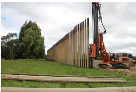
Figure 16: Sheet pile installation with RG 19T
