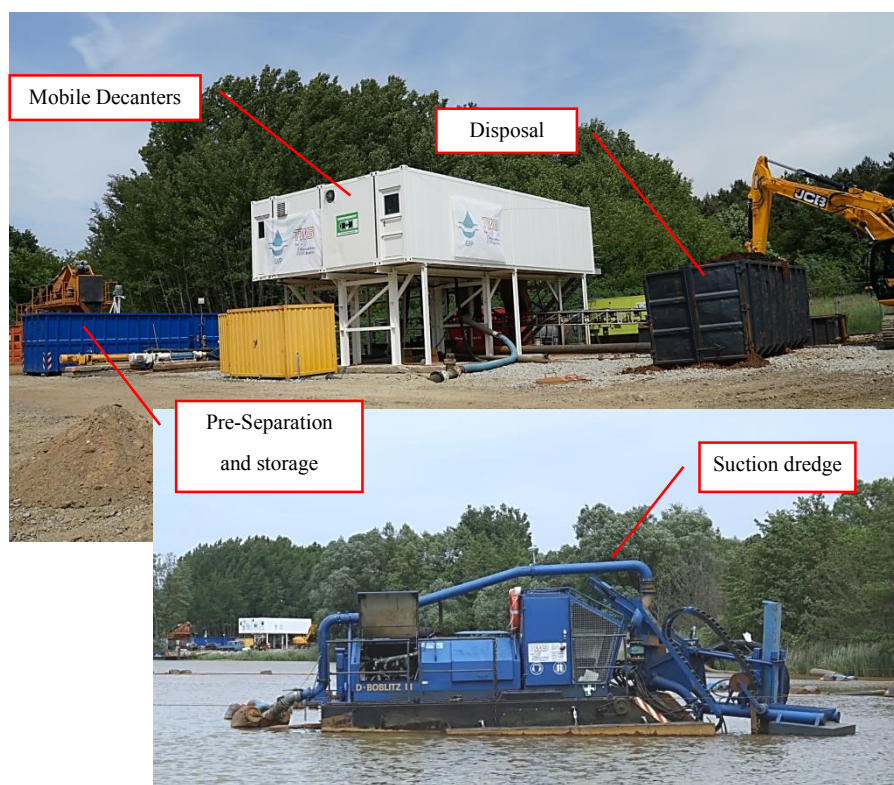
Figure 6 Desludging the Bühlow preimpoundment basin
