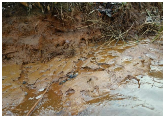
Figure 6 Evidence of groundwater influx on the right bank..
