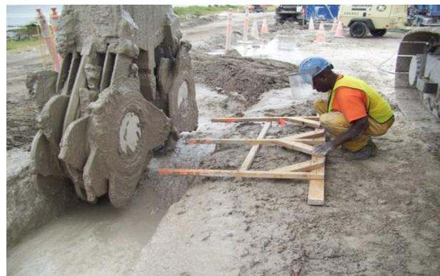
*Figure 12: BCM 5 CSM Cutter wheel assembly*
