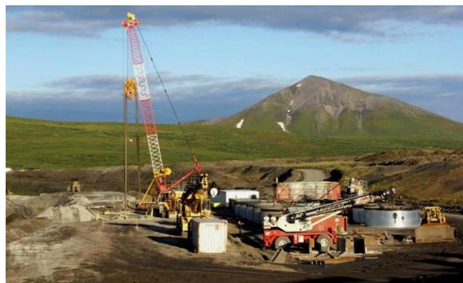
*Figure 14: Cut-off wall installation with cutter BC 40*
