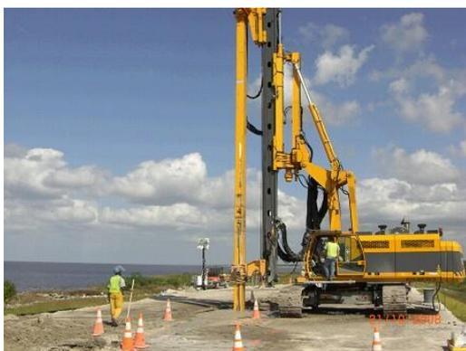
*Figure 11: CSM installation with RG 25 S*
