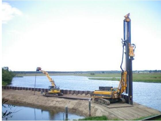
**Figure 15:** Construction of a ship lock near *Quitzebel*, Germany. Sheet pile installation with RTG RG 19T and Top Vibrator MR 105 V
