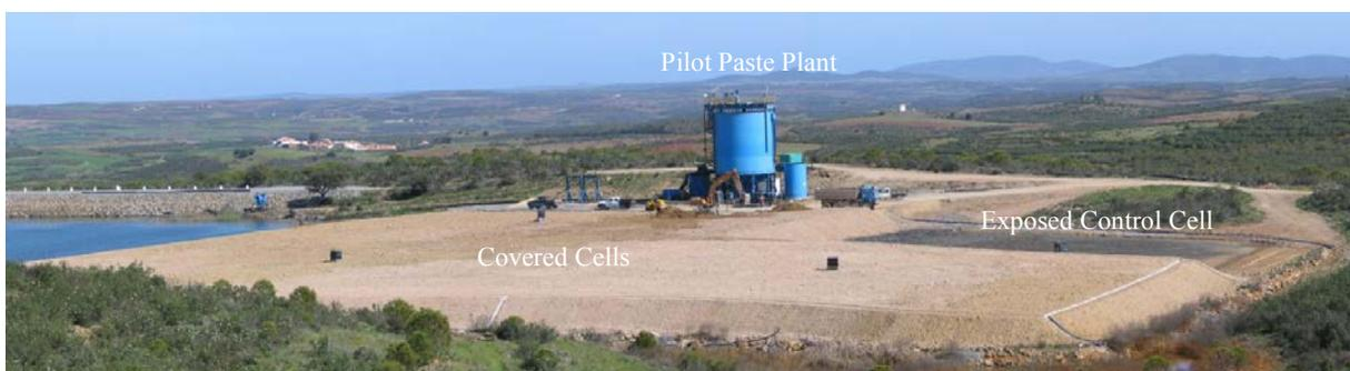
*Figure 3 Paste Trial after Construction.*
