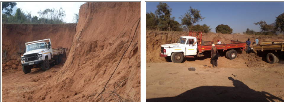
Figure 3 Sand mining operation at Dopeni village
