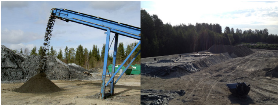
Figure 1 Mixing experiment and construction of a pilot sealing layer, Boden, Sweden 2014.
