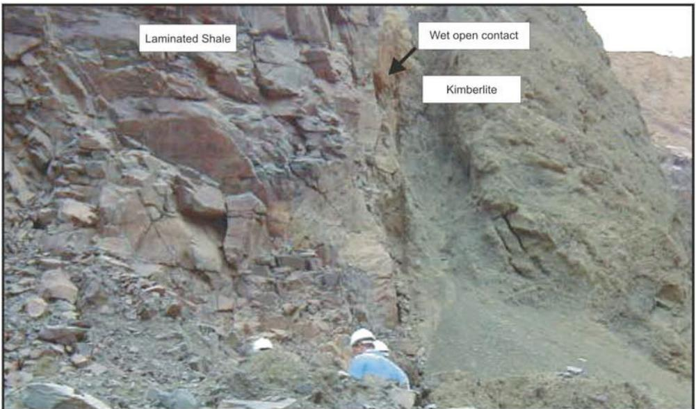
Figure 6 Jwaneng Mine Zone of Relaxation and wet kimberlite contact (crater)
