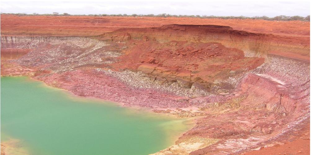
*Photograph 1: Circular failure in saturated, extremely weathered Archean rock*
