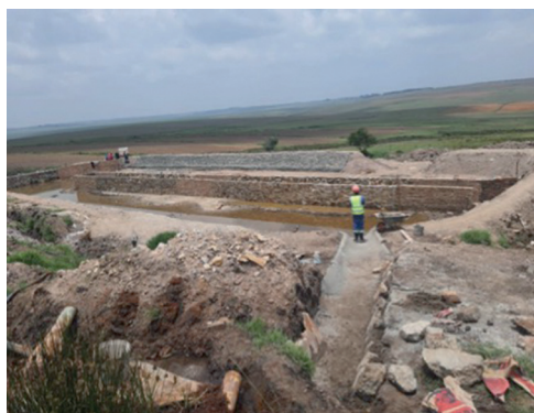
Figure 3 Refurbishment of the first pond (RAPS 1) (left) and compost mixed with limestone in RAPS 1 (right).
