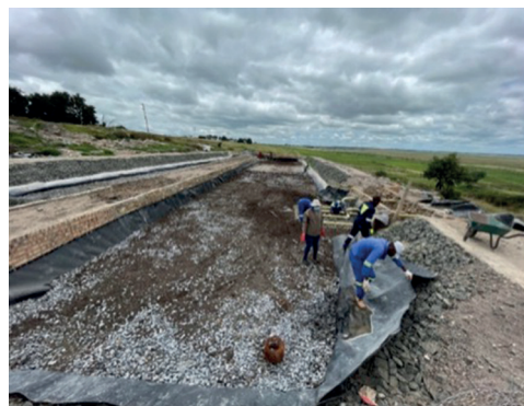
Figure 3 Refurbishment of the first pond (RAPS 1) (left) and compost mixed with limestone in RAPS 1 (right).
