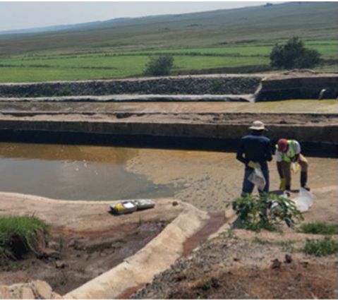
Figure 4 An overview of RAPS 1 showing channelled inlet water, ponded mine water under treatment and a berm in the center (for increasing retention time).
