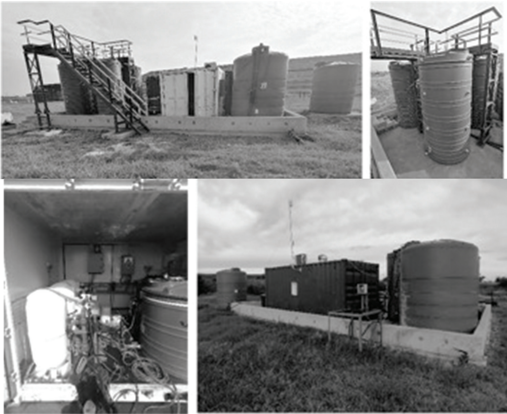
Figure 2 Semi-active pump and treat plant implemented at site B, located in the North West province of South Africa.
