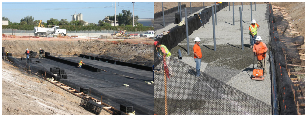
Figure 1 Example construction of a subsurface GBR™.
