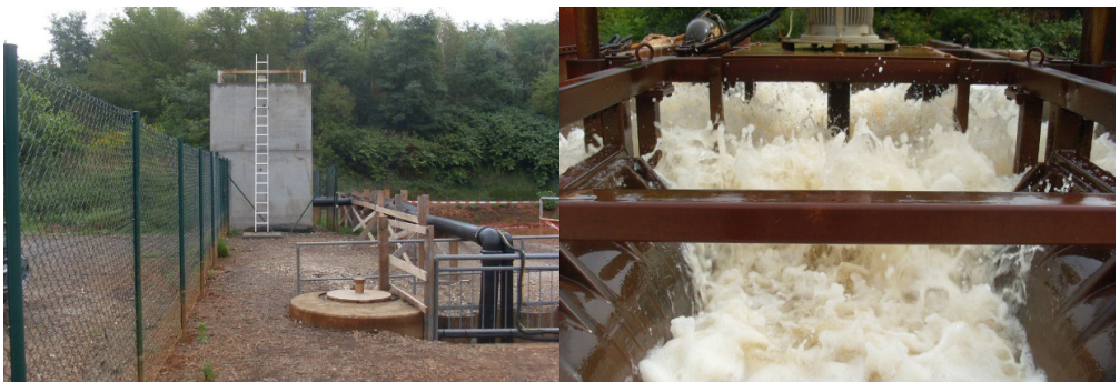
Figure 1 View on the pre-aeration tank (left side) and the surface aerator in operation (right side).
