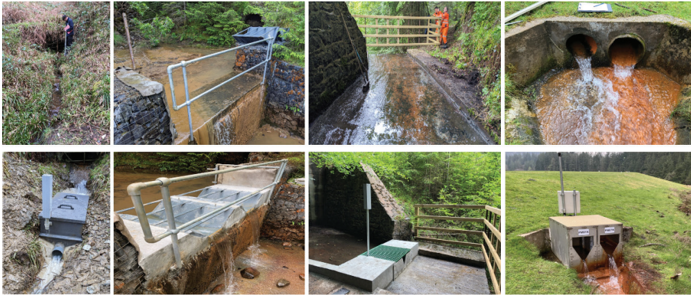
Figure 4 Parc Mine flow monitoring structures
