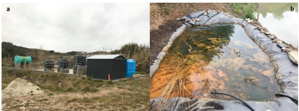
Figure 2 Pictures of on-site pilot (a: pozzolana bio-filter and iron oxi-hydroxide settling tank, b: finishing pond).
