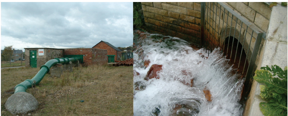
Figure 2 Photographs of Page Bank, former pumping station left, and gravity discharge right
