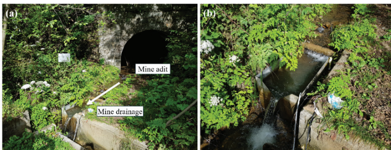
Figure 1 (a) Overview of a site at G mine with a single adit discharging mine drainage, and (b) a detailed view of the mine drainage.
