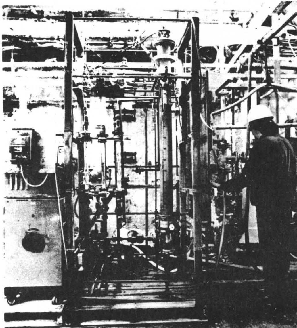
Figure 8. FBE-unit removing mercury from a brine stream
